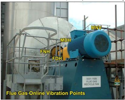
The above Photo illustrates the position of the fixed online vibration sensors that are fitted to the fan and motor (i.e. MNV = Motor Non Drive End Bearing Vertical).
